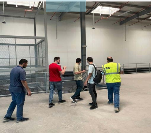
Construction site visit to a warehouse building under construction on October 9, 2021.
